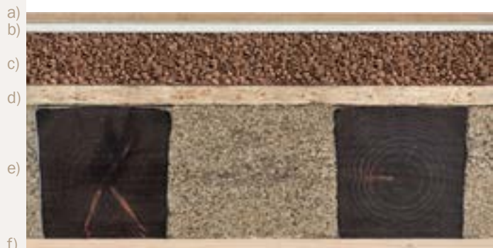
Wooden beam ceiling
