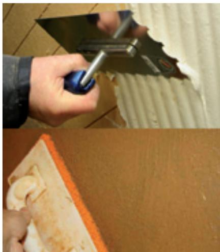
If the **UdiMULTIGRUND**® is combed with a toothed trowel, a **UdiLOAM**® Loam plaster or mortar can also be applied.
