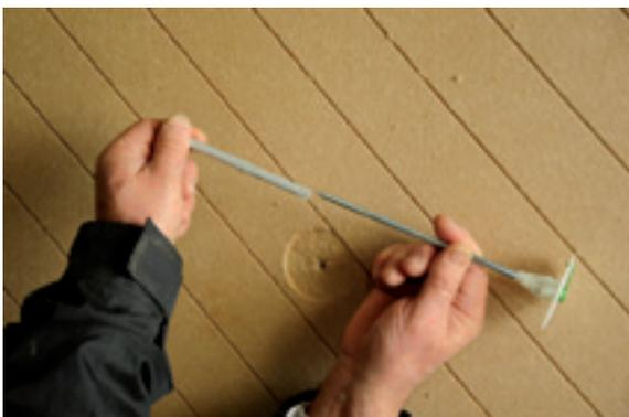
The **UdiASSEMBLY**® SDM (adjustable fixing - Masonry) is supplied in two parts. The screw should initially be screwed into the plug with approximately two turns.
