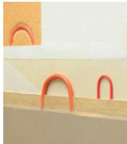
Wall heating systems can also be installed onto the plaster-finished surface. These should be fixed securely to the substrate.
