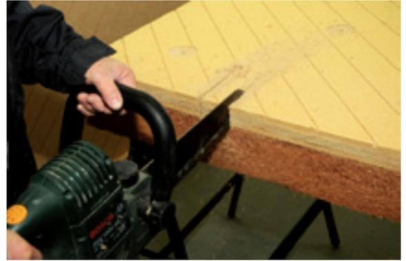
Using an electric 'alligator' saw only cut away the plaster-bearing layer.
