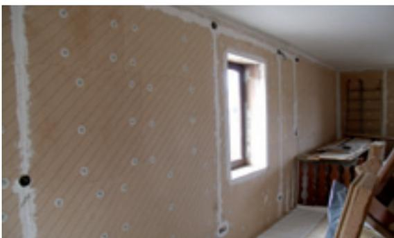
Horizontal or vertical grooves can be cut into the boards for electrical cables. Alternatively, the cable can be affixed to the substrate underneath the insulation layer.
