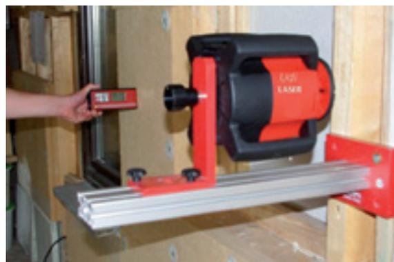
Once all the fixings are correctly installed these can then be adjusted one after the other. We recommend that you use a rotating laser or alternatively use a long spirit level. It is only possible to work wall-for-wall i.e. once a whole wall is correctly adjusted, the installation of the boards on the next wall can begin.
