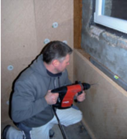
A minimum of 8 adjustable fixings should be used per *Udi*RECO® wood-fibre insulation board.
