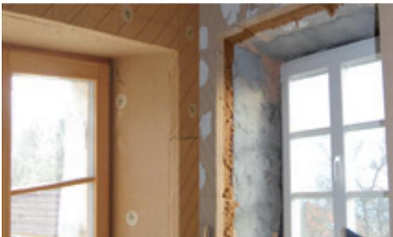
All apertures, such as windows and doors, must then be cladded with reveal insulation boards.
