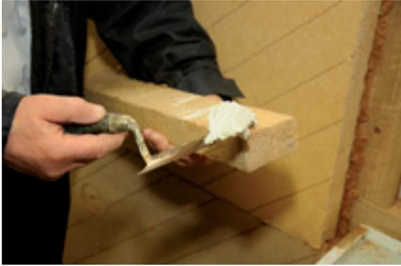
The **UdiUNGER-DIFFUTHERM® L** Reveal insulation board is stuck to the **UdiRECO®** Insulation board using our solvent-free **UdiSPECIAL ADHESIVE®**.
