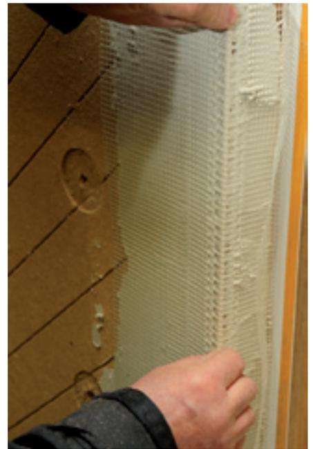
Then embed the **UdiREINFORCEMENT®** Corner Protection Profile. Ensure it is plumb.
