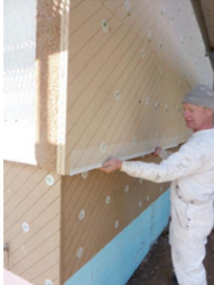
After successfully adjusting the *UdiRECO*® insulation boards, the *UdiBASE*® Slot-in profile is inserted and bonded flush using render to fill the gaps.
