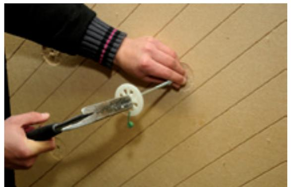
The fixing should then be skilfully inserted into the hole and carefully hammered home until the fixing head is a minimum of 30 mm from the board surface.
