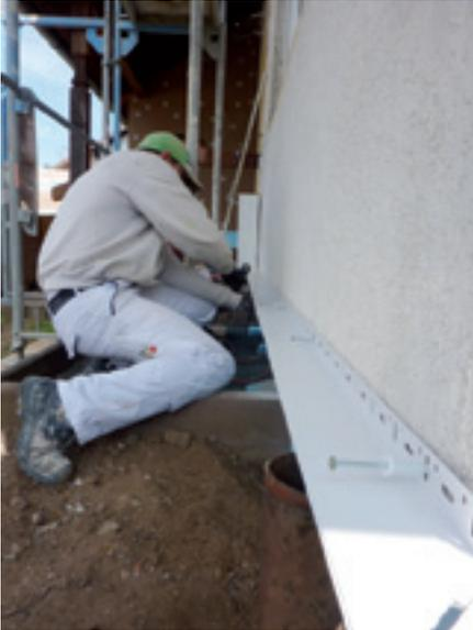
Firstly, the *UdiBASE*® wall connection profile is fixed flush and level on to the substrate.
