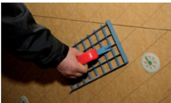
Uneven joint edges should be smoothed using a grid plane/trowel (picture) or an electric disc-type sander. This helps to ensure a uniform coating thickness when applying the reinforcement render.
