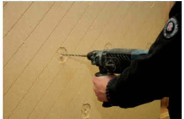
Take care that the fibres in the drill hole have been removed properly. To achieve this simply repeat the drilling procedure in the upper layer of the board.
