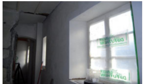
The self-adhesive *Udi*REINFORCEMENT® Render Edging Strip **INSIDE** is stuck to the frame and coated with *Udi*MULTIGRUND® to provide a neat, finished plastered edge.
