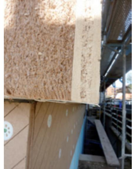
This forms a neat and thermally efficient plinth/lower edge finish with a drip edge to protect against the ingress of moisture, rain and snow.
