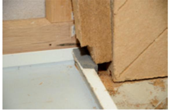
Beforehand, the **UdiJOINTING TAPE®** should be installed and the reveal insulation board disengaged.
