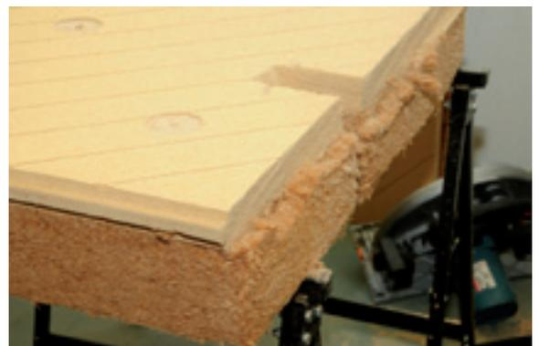
The picture shows the protruding flexible layer e.g. for connections to walls, roof areas. This ensures a good contact to the insulation layer.
