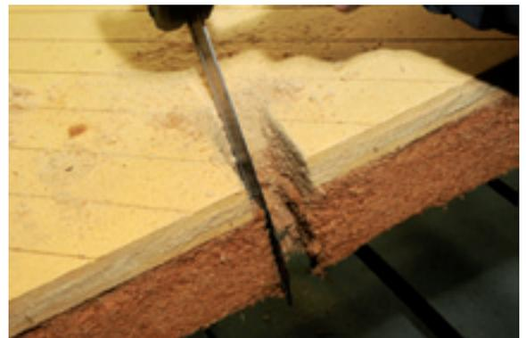
Cutting the lower, flexible layer allowing an excess (projection above the plaster-bearing layer).
