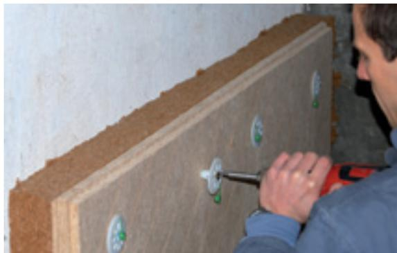
By exerting a direct influence on the moisture level, the capillary-active insulation system **UdiIN RECO®** inhibits problems with moisture which may lead to building damage. With this system, a simple and effective solution has been developed which meets the requirements for energy saving and contributes to a healthy room climate. It can be used for any application from thin, half-timbered wall constructions to thick castle walls.
