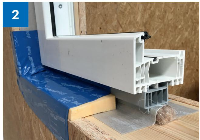
> Example of gradient with an insulating wedge.
