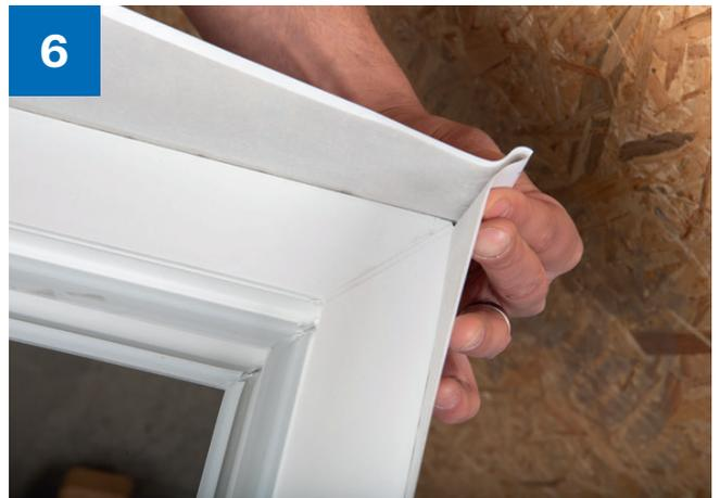
> Squeeze loop together and press on well.
