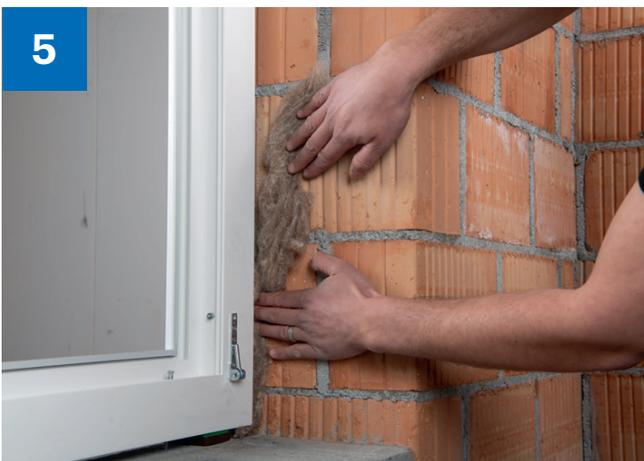
5 > Insulate joints ensuring there are no cavities.
