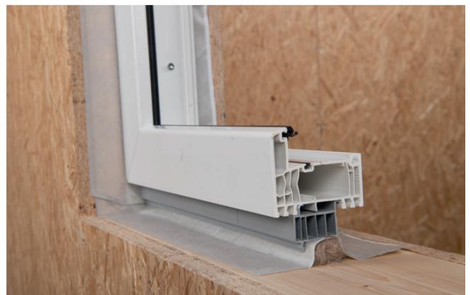
> Stick Ampacoll® Fenax DS for alternating bonding to the inside and outside of the window frame, then press on well. Create corner loops: approx.  $1.5 \times$  joint width. Insulate joints ensuring there are no cavities. Left: without window connection profile (FBA). Right: with FBA. **Note:** Observe the design of the window sill base, see pages 17–19 second sealing layer / window sill base.
