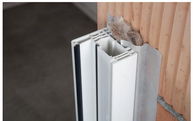
> Stick Ampacoll® Fenax DS for alternating bonding to the inside and outside of the window frame, then press on well. Create corner loops: approx.  $1.5 \times$  joint width. Insulate joints ensuring there are no cavities. Create relief loops.
