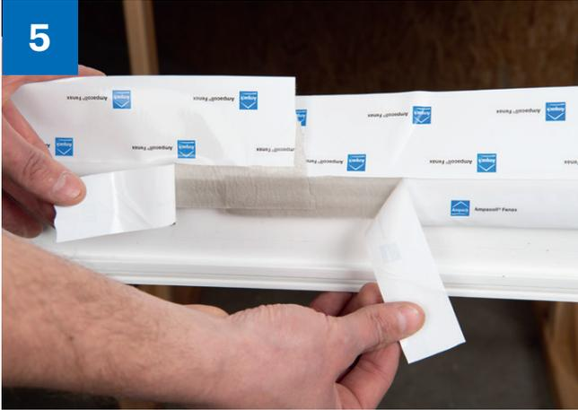
> Where the sealing foils meet, make sure that the ends overlap and that the connection is airtight, windtight and impermeable to driving rain.
