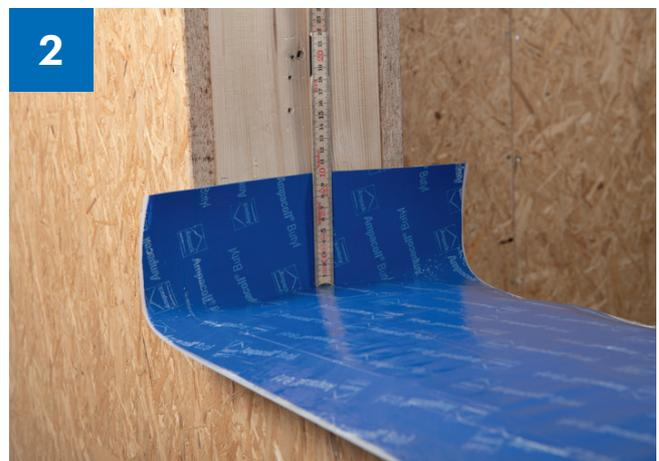
> Cut Ampacoll® Sillskin to length allowing for lateral overlap and press on. Side overlap: DE  $\geq 10$  cm; AT  $\geq 6$  cm.
