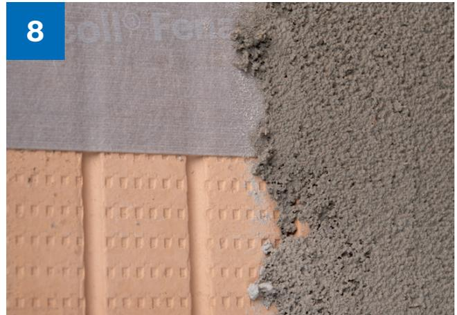
> The airtight layer is created by plastering over the tape.
