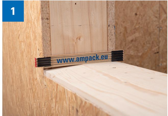
> Creation of  $\geq 5^\circ$  gradient in the wall element or installation of e.g. wood or insulation wedge.
