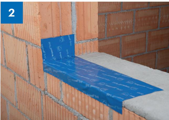
> If Ampacoll® Sillskin reaches into the plaster area of the façade, cut out any lateral overlap. Now the window frame can be positioned and mounted in the wall opening.
