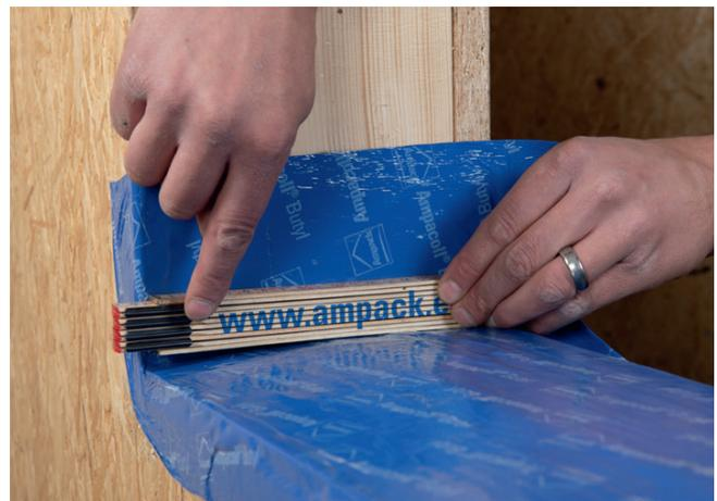
> Schematic diagram for timber construction (left) and application example of Ampacoll® Sillskin (right). Side overlap: DE ≥ 10 cm; AT ≥ 6 cm.
