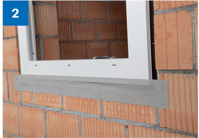
2 > Start at the bottom, then the sides, then the top (water flow)
