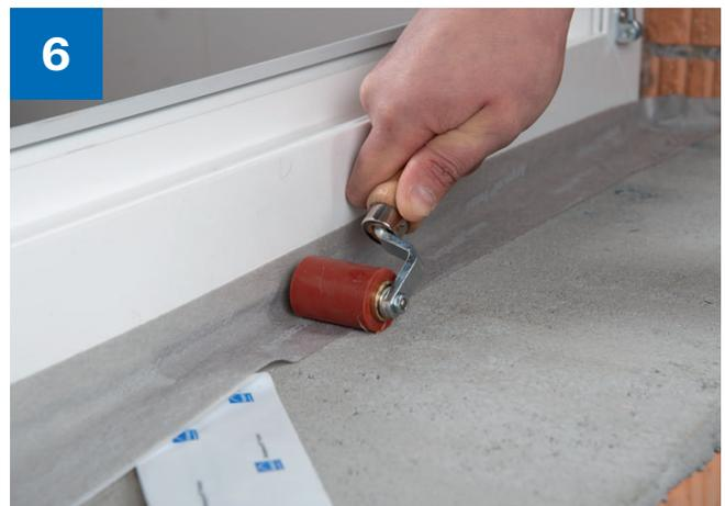
6 > Start bonding at the bottom. Press on well.
