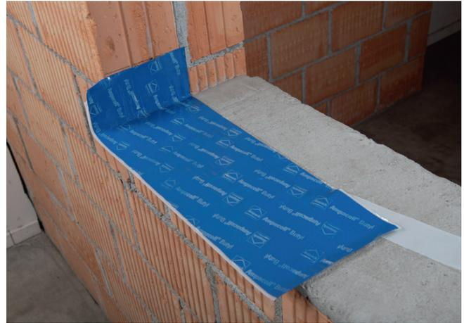
> Mark the position in the reveal. Cut Ampacoll® Sillskin to length allowing for lateral overlap, then firmly press on the adhesive tape. Side overlap: DE  $\geq$  10 cm; AT  $\geq$  6 cm.
