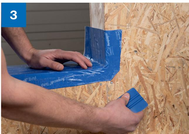
> Thanks to its high extensibility, Ampacoll® Sillskin can effortlessly be installed in the corners. The result is a continuous one-piece cover.
