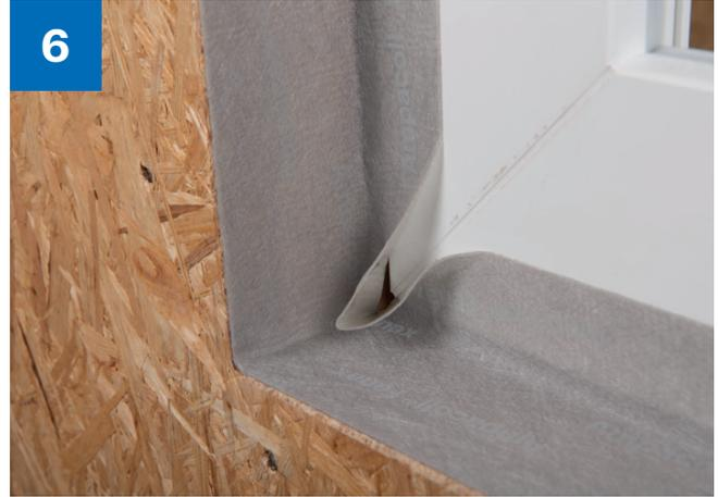
> **Tip:** Circumferential installation of Ampacoll® Fenax after window installation (without incision and in a single pass). The corner can be made without cutting by creating an inverted pleat.
