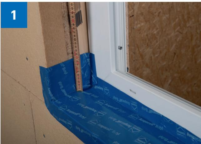
> After the window has been installed, the window sill base is stuck to the outside of the window frames with Ampacoll® Sillskin.
