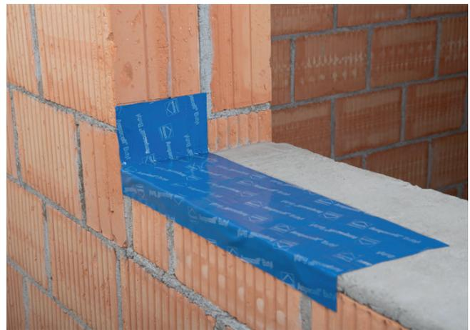
> Schematic diagram for solid construction (left) and application example of Ampacoll® Sillskin (right). Side overlap: DE  $\geq$  10 cm; AT  $\geq$  6 cm. If Ampacoll® Sillskin reaches into the plaster area of the façade, cut out any lateral overlap.
