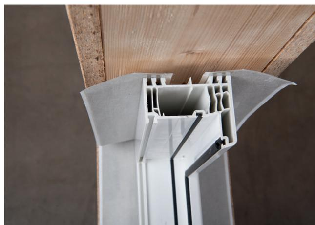
**Example:** On the left, the two prefabricated Fenax skirts. On the right, central installation in wooden frame wall. Insulate joints ensuring there are no cavities. Apply the Ampacoll® Fenax adhesive tapes tension-free or with a relief loop.
