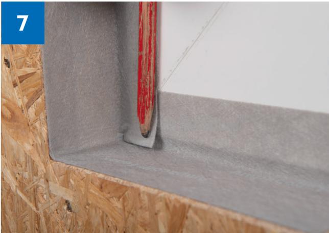
> Rub the inverted pleat together well and then fold it down (water flow).
