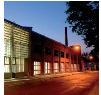
Reconstruction of the old weaving mill in Fulda, following a fire: Interior insulation with Ytong Multipor mineral insulating system
