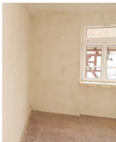
The characteristics of the room were maintained perfectly.
