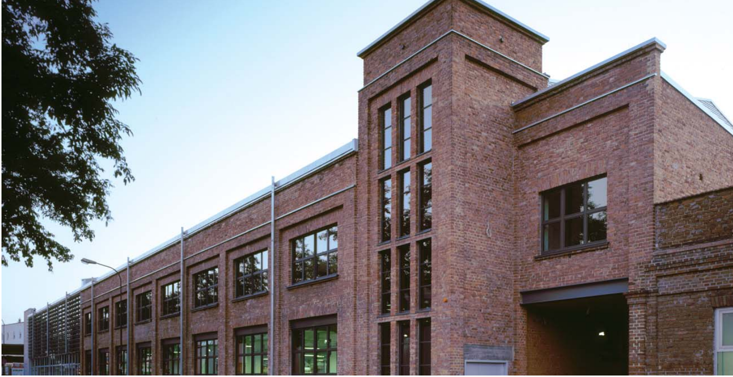
Old weaving mill in Fulda, damaged highly by fire, completely rebuilt
