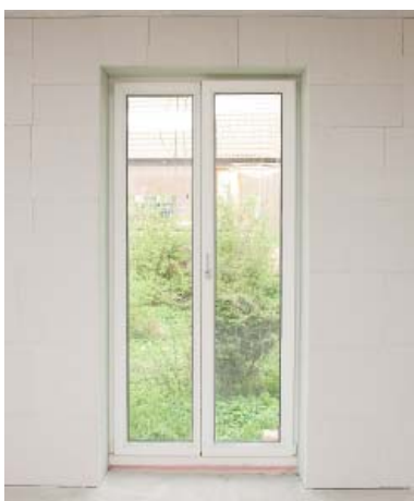
Insulating exterior walls on the inside with Ytong Multipor Mineral Insulation Boards allowed successful conversion of a nearly 80 year old farmhouse.
