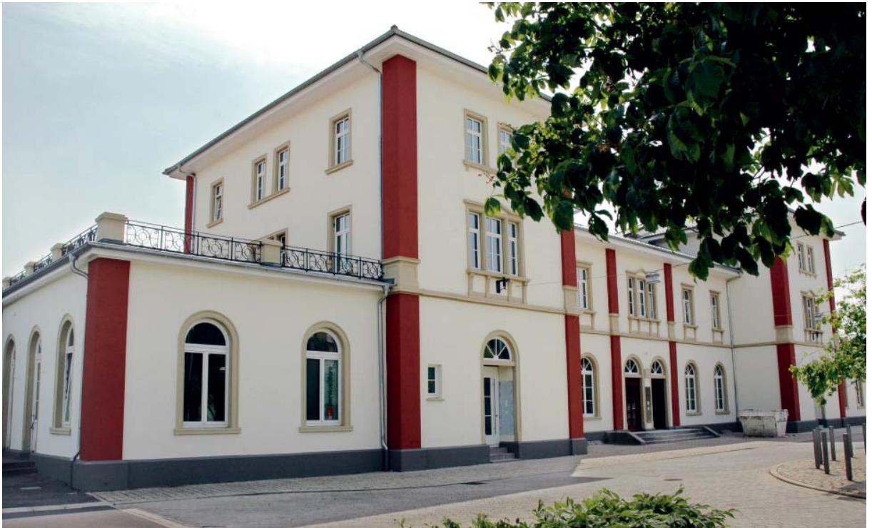
Ytong Multipor as interior insulation allowed the appearance of this historical building to be maintained while improving the insulating value to nearly that of a "standard passive building".
