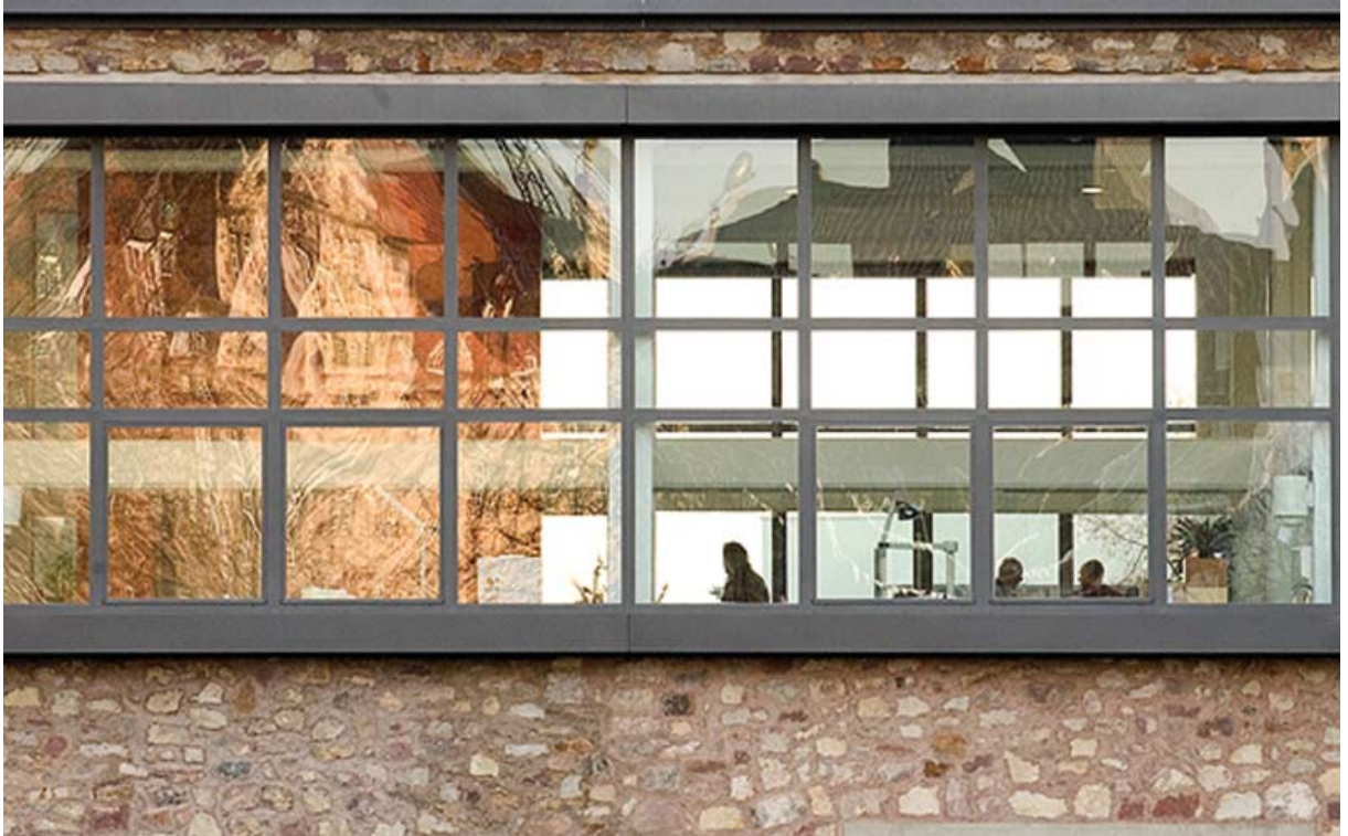
Renthof, Kassel – modern thermal insulation on historical building
