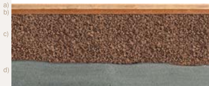
Solid ceiling with fibreboard
