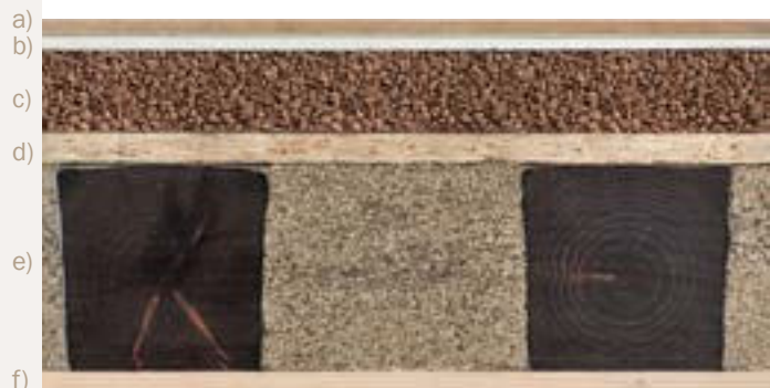
Wooden beam ceiling
