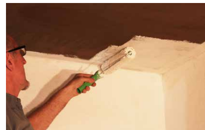
Coating with clay plaster and clay paint
