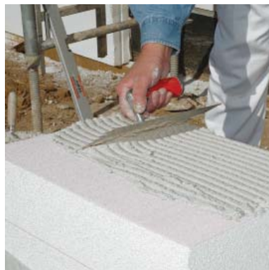
Apply over full surface with toothed trowel (10 or 12 mm teeth) results in adhesive surface of at least 70%.
