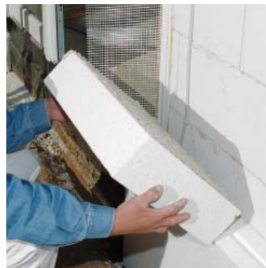
Base height of light mortar approx. 8–10 mm. This allows irregularities up to 5 mm in the subsurface to be compensated.
