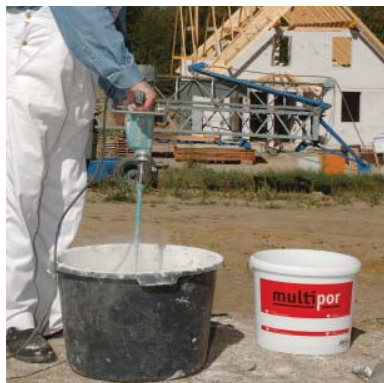
Mixing light mortar. 20 kg mixed with 8 l of water (mark on measuring bucket) yields approx. 30 l of adhesive mortar.
