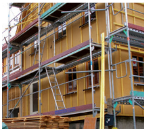
UdiTOP ® – summertime heat shielding and windproofing combined in one product
