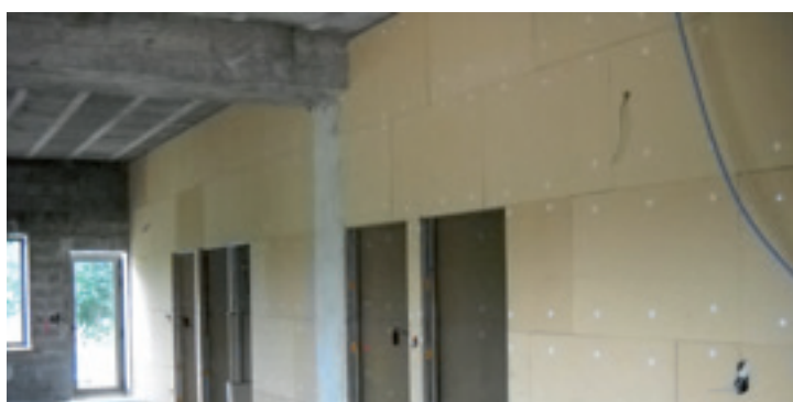
UdiCLIMATE ® is applicable as an underside, roof insulation board or dry lining layer for walls
