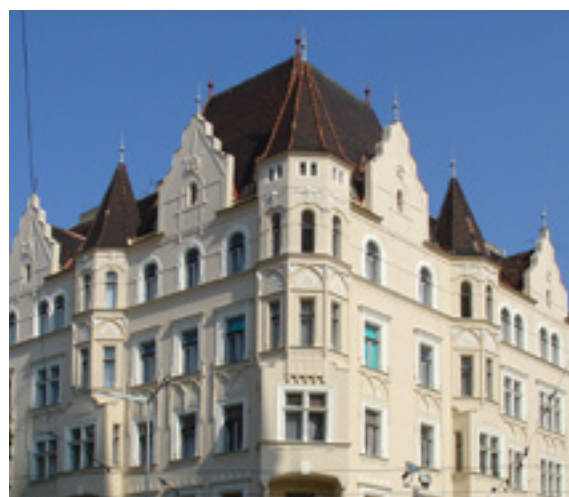
This sight of this beautiful façade has been retained thanks to UdiIN 2CM ® internal insulation
