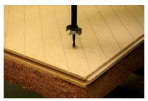
Countersinking provides a neater result but is not absolutely necessary. Recess depth: max. 3 mm.
