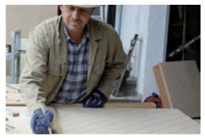
By using a template it is easier to exactly mark the position of the hole(s) required. For a perfect result the surface can also be countersunk to receive the fixing head disc.
