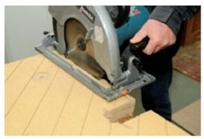
Now cut approximately 1-2 cm from the plaster-bearing layer to provide a snug fit to adjacent building elements e.g. floors, soffits, joists etc
