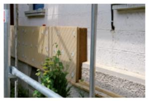
Cut-outs for large protrusions should be performed before installing.
