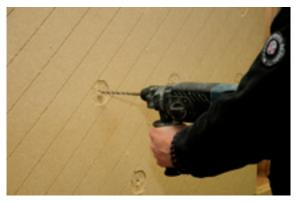
Take care that the fibres in the drill hole have been removed properly. To achieve this simply repeat the drilling procedure in the upper layer of the board.
