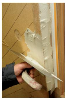
Apply sufficient UdiFOUNDATION COAT®
