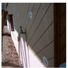
Ready installed insulation layer. The water tap can be reused.
