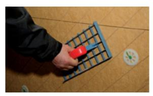
Uneven joint edges should be smoothed using a grid plane/trowel (picture) or an electric disc-type sander. This helps to ensure a uniform coating thickness when applying the reinforcement render.
