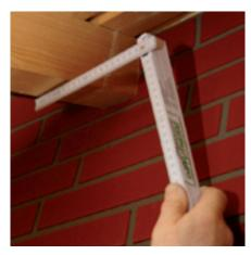
Take measurements. Cut-outs must be made for visible rafters.
