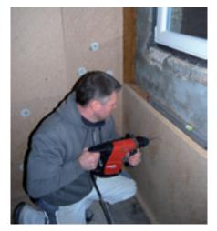
A minimum of 8 adjustable fixings should be used per Udi**RECO**<sup>®</sup> wood-fibre insulation board.
