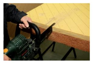
Using an electric 'alligator' saw only cut away the plaster-bearing layer.
