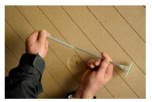
The *Udi***ASSEMBLY**<sup>®</sup> SDM (adjustable fixing - Masonry) is supplied in two parts. The screw should initially be screwed into the plug with approximately two turns.
