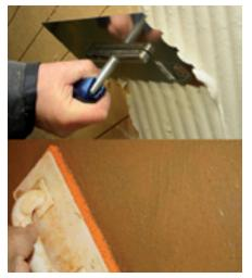
If the *Udi***MULTIGRUND**<sup>°</sup> is combed with a toothed trowel, a *Udi***LOAM**<sup>°</sup> Loam plaster or mortar can also be applied.
