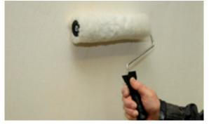
Roll on the ready-to-use render primer in accordance with the particular colour shade and system requirements
