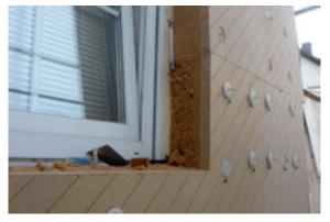
The picture shows an exact, countersunk fixing hole layout. 8 adjustable fixings are required per square metre/ insulation board.
