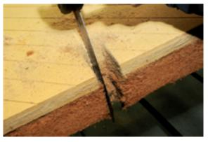
Cutting the lower, flexible layer allowing an excess (projection above the plaster-bearing layer).
