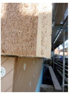
This forms a neat and thermally efficient plinth/lower edge finish with a drip edge to protect against the ingress of moisture, rain and snow.
