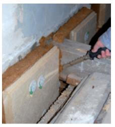
Joints should be filled with wood-fibre, waste material so that there are no gaps.
