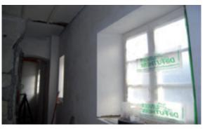
The self-adhesive *Udi***REINFORCEMENT**<sup>°</sup> **Render Edging Strip INSIDE** is stuck to the frame and coated with *Udi***MULTIGRUND**<sup>°</sup> to provide a neat, finished plastered edge.
