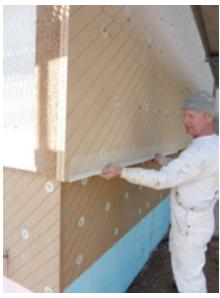
After successfully adjusting the *Udi***RECO**<sup>®</sup> ilnsulation boards, the *Udi***BASE**<sup>®</sup> Slot-in profile is inserted and bonded flush using render to fill the gaps.
