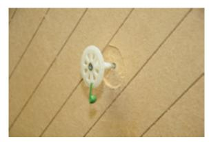
Ensure a clearance of approx. 30 mm to the board surface.
