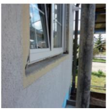
Correctly measure the required window sill length beforehand.
