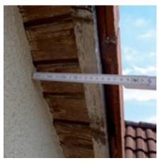
Check roof overhang. This will be reduced according to the respective insulation thickness.
