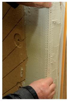
Then embed the *Udi***REINFORCEMENT**<sup>®</sup> Corner Protection Profile. Ensure it is plumb.
