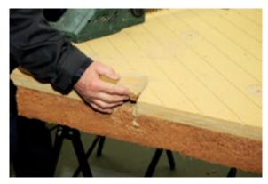
Removing the upper, plaster-bearing layer.
