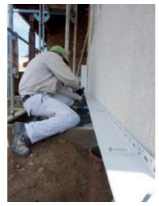
Firstly, the *Udi***BASE**<sup>®</sup> wall connection profile is fixed flush and level on to the substrate.
