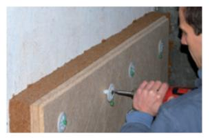
By exerting a direct influence on the moisture level, the capillary-active insulation system UdiIN RECO<sup>®</sup> inhibits problems with moisture which may lead to building damage. With this system, a simple and effective solution has been developed which meets the requirements for energy saving and contributes to a healthy room climate. It can be used for any application from thin, half-timbered wall constructions to thick castle walls.
