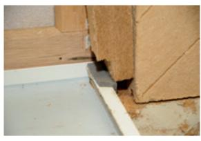
Beforehand, the *Udi***JOINTING TAPE**<sup>®</sup> should be installed and the reveal insulation board disengaged.
