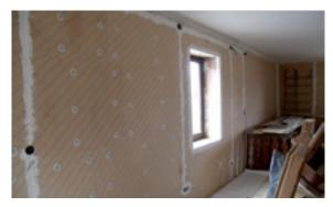
Horizontal or vertical grooves can be cut into the boards for electrical cables. Alternatively, the cable can be affixed to the substrate underneath the insulation layer.
