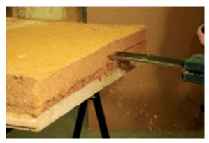
Large unevenness's or protrusions can be compensated for by cutting away a section of the flexible insulation layer.
