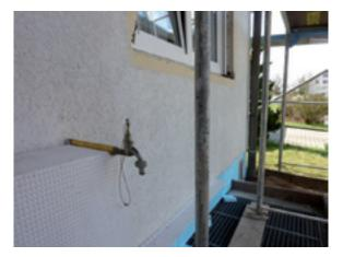
Select the water tap extension according to the insulation thickness.
