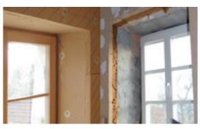
All apertures, such as windows and doors, must then be cladded with reveal insulation boards.
