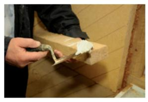
The *Udi***UNGER-DIFFUTHERM**<sup>®</sup> L Reveal insulation board is stuck to the *Udi***RECO**<sup>®</sup> Insulation board using our solvent-free *Udi***SPECIAL ADHESIVE**<sup>®</sup>.
