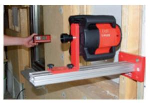
Once all the fixings are correctly installed these can then be adjusted one after the other. We recommend that you use a rotating laser or alternatively use a long spirit level. It is only possible to work wall-for-wall i.e. once a whole wall is correctly adjusted, the installation of the boards on the next wall can begin.
