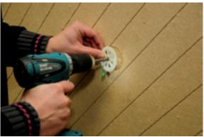
Hold the fixing head securely when screwing in to avoid it rotating with the screw. The fixing head sits perfectly when it is flush with the surface. To ensure that the fixing is thermally decoupled, always insert the green sealing cap into the aperture provided
