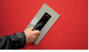
The surface is then structured by hand or else using a plastering machine with an adjustable flow rate. The finished structure must have a uniform appearance but can vary slightly due to the craftsmanship individual workers.
