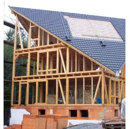
In terms of structural physics, this construction represents the most up-todate technical standards. Almost all of the worst constructional mistakes caused by the build up of condensation can be eliminated. The stabilising effects of the natural moisture balance reduce the intrinsic movements of the timber.
