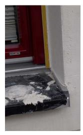
*Udi***REINFORCEMENT**® **Corner Strengthening Mesh** is bedded-in above and below the corners of window and door openings. *Udi***REINFORCEMENT**® **3D Corner Strengthening Mesh 90 Degree** is also bedded-in but in this case only above the openings. The *Udi***FOUNDATION COAT**® should then be smoothed flat with a stainless steel trowel (drying time 1 mm = 1 day). Cut edges (e.g. in the vicinity of scaffold anchors) must have a double layer of reinforcing mesh.
