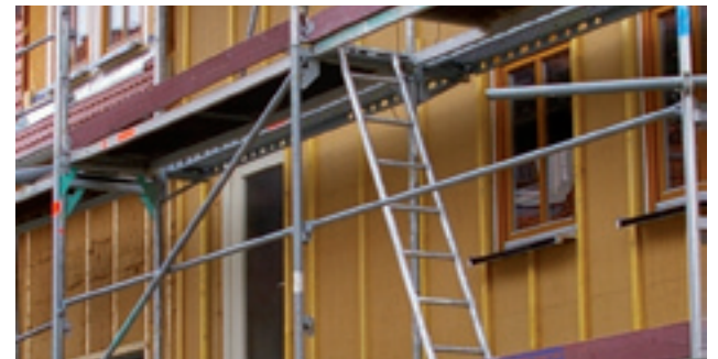
Application: The external cladding of rear-ventilated façades directly onto timber-frame constructions; for use with solid timber elements and on masonry walls behind the curtain walls.
