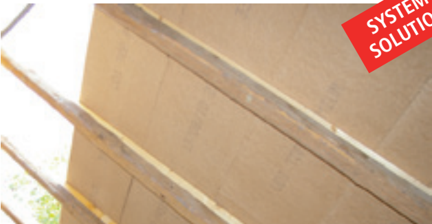
Application: Full-surface, wind-tight, sark boards in accordance with the new European standard DIN EN 14964 and the German Roofing Industry Association standards.
