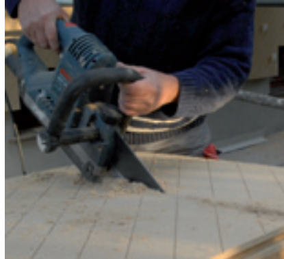
The insulation boards can be cut to size using an electric saw
