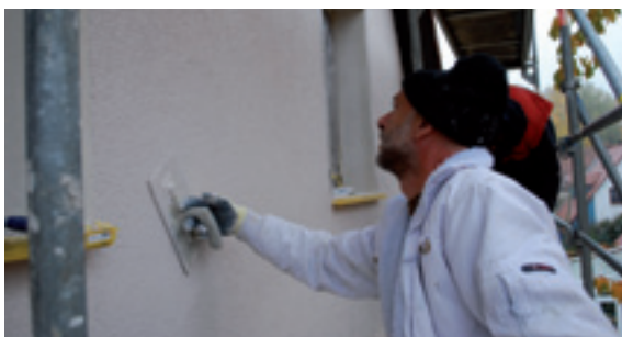
Specially matched structured fine renders from the Unger range are used as a finishing coat
