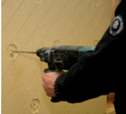
Drill a hole in the substrate to position the fixing
