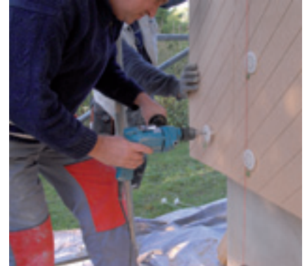
The adjustable fixing both secures and levels the insulation board
