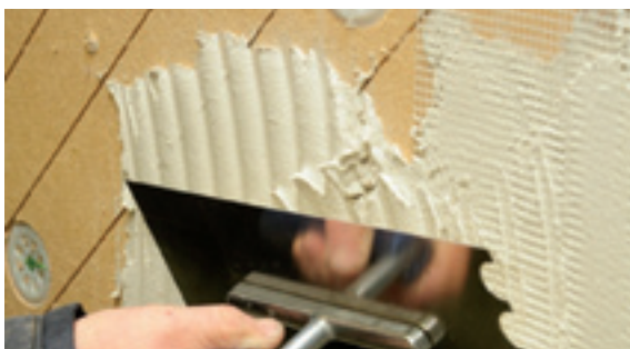
UdiFOUNDATION COAT® with a crack-bridging layer of UdiREINFORCEMENT® Strengthening mesh is applied as the first coat
