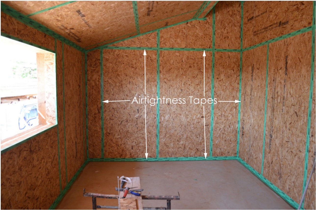
(Green airtightness tape in use)
