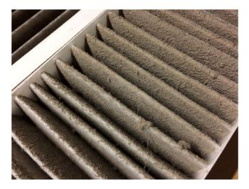
After 3 months the air filters can be really filthy, especially if you live in an urban environment or near roads. During the cold months the intake filter can become full of black mould and if left this mould will inevitably start growing in the filter and allowing spores to be blown in to your home. This can have implications to your respiratory health.
