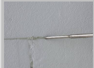
Fig. 14 Fill in joint gaps less than 5mm with system foam.
