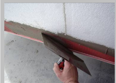
Step 16 Smooth out the mortar.
