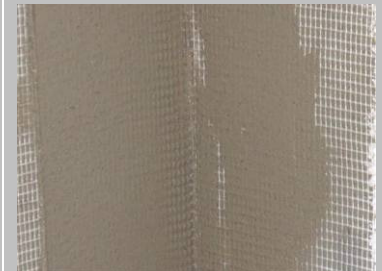
Step 2 Apply additional reinforcing mesh (min. 200mm wide) around internal corners in a tight coat of bonding mortar.
