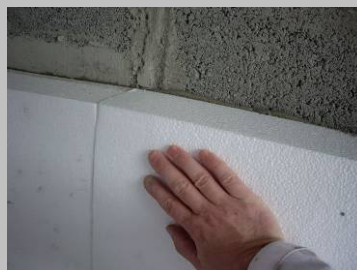
Fig. 7 Butt the boards tightly together and ensure the surfaces are flush.
