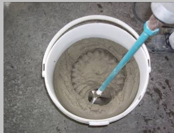
Fig. 1 Sprinkle the dry powder adhesive into clean water. Mix with an electric hand mixer at slow speed setting to a smooth, workable mortar.
