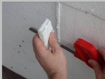
Fig. 13 Cut back the excess as slightly proud of the surface.
