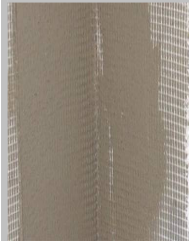
Fig 4 Apply additional reinforcing mesh (min. 200mm wide) around internal corners in a tight coat of bonding mortar
