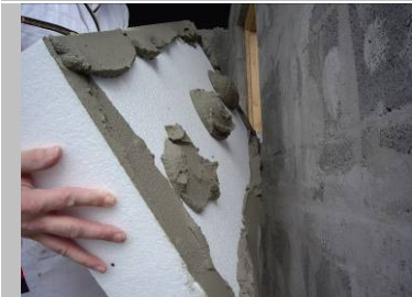
Fig. 6 Place the board on to the wall and “wobble” it into position.
