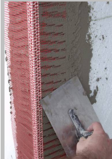
Step 6 Place the angle bead in position level and smooth out the mesh.
