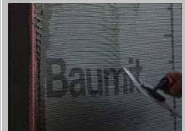
Step 6 Lightly trowel over the mesh surface from the middle outwards to avoid creasing.
