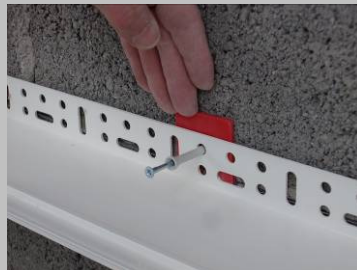
Step 3 Place a packer between the substrate and the L section and push it down onto the fixing shaft until it clicks.
