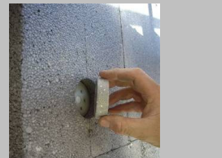
Step 8 Place cap on to the head of the fixing, push in.
