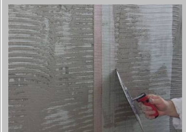
Step 8 Overlap the next mesh sheet (min. 100 mm) onto the edge and lightly smooth out with the trowel. Then apply a little more material as necessary to cover the mesh leaving it just under the surface.
