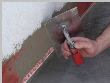
Step 15 Trowel the mesh into the base coat mortar.
