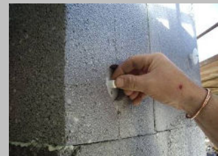
Step 6 Remove the drill and place a STR U plug into the shaft void so stop thermal bridging.
