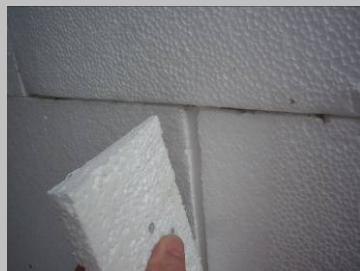
Fig. 11 Cut a wedge of insulation material.
