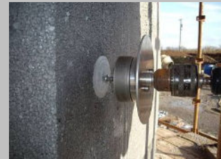
Step 4 Using the STRU drill attachment placed on the head of the fixing, drill the fixing into place.
