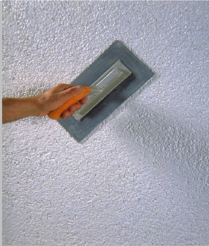
Step 5 Using a plastic float working in small circular motions texture the surface to a uniform finish.
