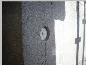
Step 4 Fixing will be counter sunk to 15mm when the drill locks.
