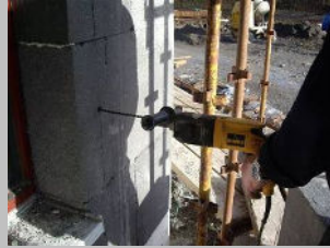
Step 1 Drill Through the insulation and into the wall approx 75mm into background.
