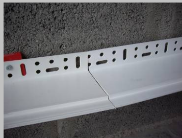
Step 5 Butt each following L-section up tight and continue until a complete wall section is finished.
