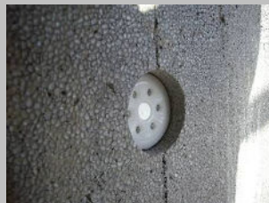
Step 7 Plug fits into shaft.
