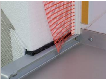
Step 5 Peel off all the yellow paper tape from the protection strip to expose the sticky surface to allow the application of polythene sheet to protect the window from mortar splashes.
