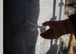
Step 2 Push the screw fixing through into the bore hole.
