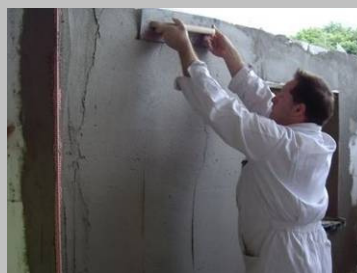
Step 3 Spray or hand apply the bonding mortar over the surface and smooth out with a trowel or plastering rule.
