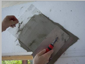
Step 1 Apply reinforcing mesh strips (min. 250 x 250mm) diagonally across the opening corners into a tight coat of bonding mortar.
