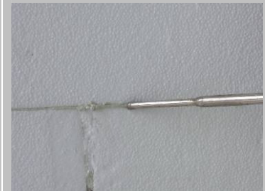
Fig. 14 Fill in joint gaps less than 5mm with system foam.
