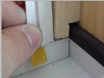
Step 3 Press the bead firmly into position, starting on the inside edge of the sill end cap and working upwards and repeat for the window real head.
