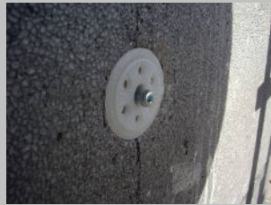
Step 3 Place the fixing head flush on the surface.
