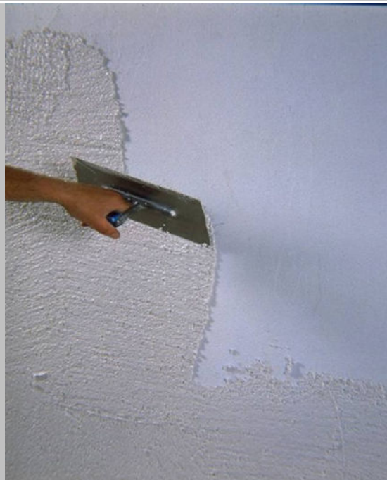
Step 4 Apply the finish to 1 grain thickness using a steel trowel.
