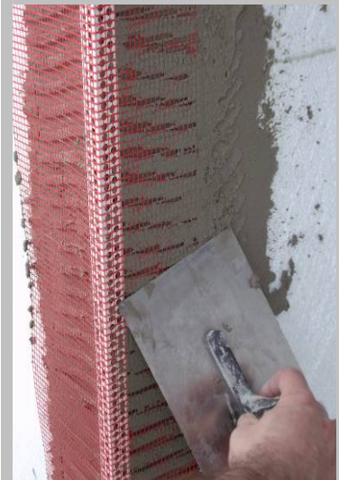
Step 6 Place the angle bead in position level and smooth out the mesh.
