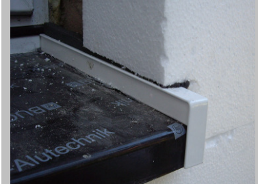
Step 2 When finished the facade insulation boards should carry past window reveal and sit 5 – 10mm in from the inside edge of the sill up-stand to accommodate the angle bead edge by at least the planned thickness of the reveal insulation (min. 30mm).
