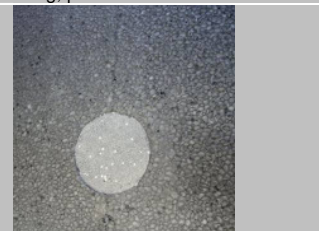
Step 8 Place cap on to the head of the fixing, push in.
