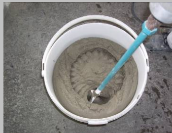
Fig. 1 Sprinkle the dry powder adhesive into clean water. Mix with an electric hand mixer at slow speed setting to a smooth, workable mortar.
