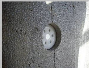
Step 7 Plug fits into shaft.
