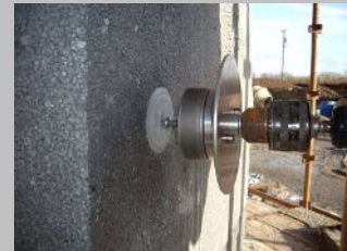
Step 4 Using the STRU drill attachment placed on the head of the fixing, drill the fixing into place.
