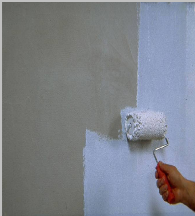
Step 2 Apply the primer over the surface using a brush or Roller. Allow to dry for 24 hours.
