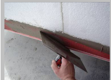
Step 16 Smooth out the mortar.
