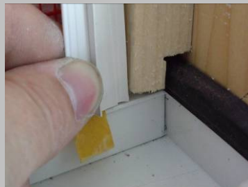
Step 3 Press the bead firmly into position, starting on the inside edge of the sill end cap and working upwards and repeat for the window real head.
