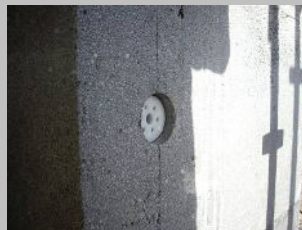
Step 4 Fixing will be counter sunk to 15mm when the drill locks.
