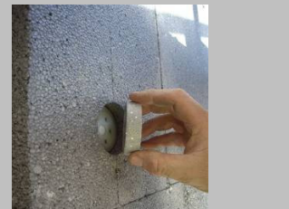
Step 8 Place cap on to the head of the fixing, push in.
