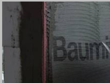
Step 5 Starting 30mm in from the corner edge of the angle bead, lay the mesh sheet lightly onto the mortar.
