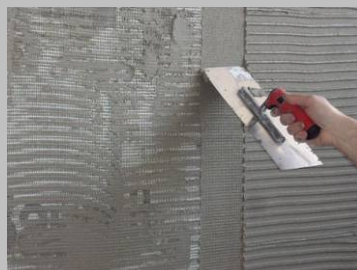
Step 7 Press the edge of the mesh sheet a little deeper into the mortar with the tip of the trowel.
