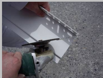
Step 7 Cut the L-section with an angle grinder or hack saw.
