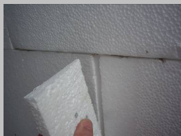
Fig. 11 Cut a wedge of insulation material.
