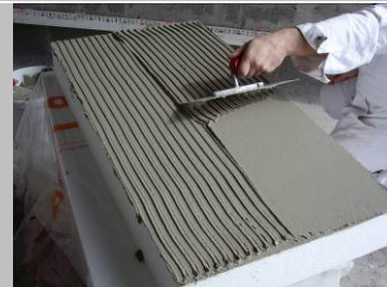
Fig. 5 Apply a full coat of adhesive mortar onto the insulation board surface and comb through with a stainless steel notched trowel.
