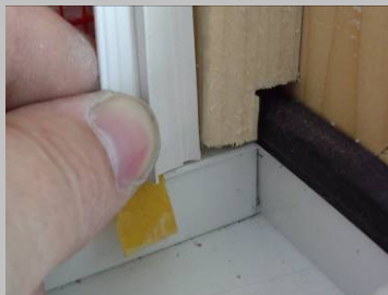
Step 3 Press the bead firmly into position, starting on the inside edge of the sill end cap and working upwards and repeat for the window real head.
