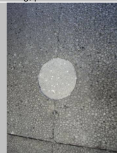
Step 10 Job Done.
