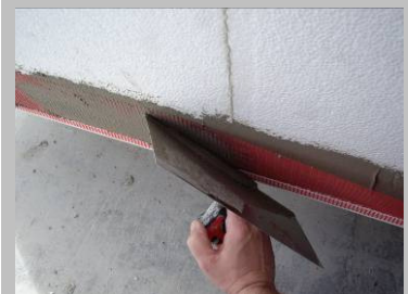
Step 16 Smooth out the mortar.
