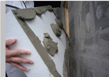
Fig. 6 Place the board on to the wall and “wiggle” it into position.
