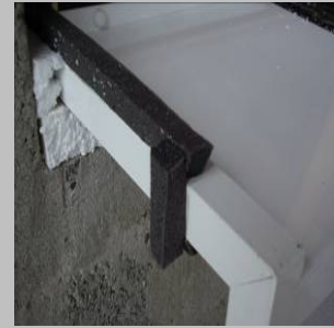
Step 4 Only apply enough band required as it will expand quickly once off the roll. Fully expanded band will be more difficult to compress later.
