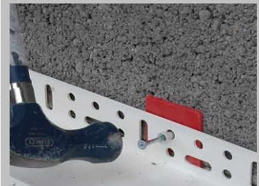
Step 6 Check the overall alignment of the L-sections and insert more packers where needed. Screw or hammer the fixing up tight.
