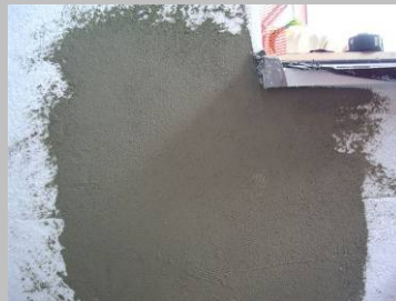
Step 1 Apply reinforcing mesh strips (min. 250 x 250mm) diagonally across the opening corners into a tight coat of bonding mortar.
