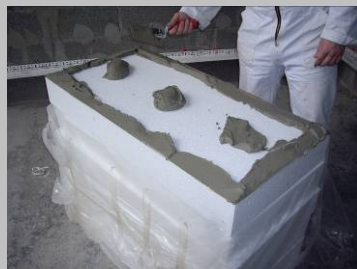
Fig. 3 Apply 3 equally spaced adhesive mortar dabs through the centre line of the insulation board and a strip around the edge.
