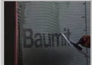
Step 6 Lightly trowel over the mesh surface from the middle outwards to avoid creasing.
