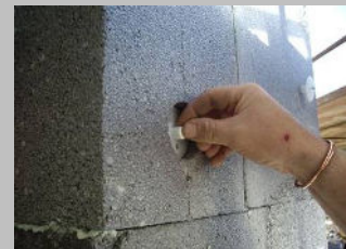
Step 6 Remove the drill and place a STR U plug into the shaft void so stop thermal bridging.
