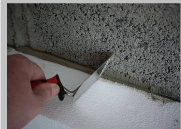
Fig. 8 Remove excess adhesive mortar
