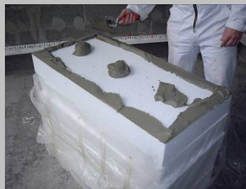
Fig. 3 Apply 3 equally spaced adhesive mortar dabs through the centre line of the insulation board and a strip around the edge.
