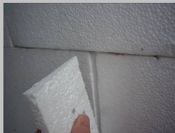
Fig. 11 Cut a wedge of insulation material.
