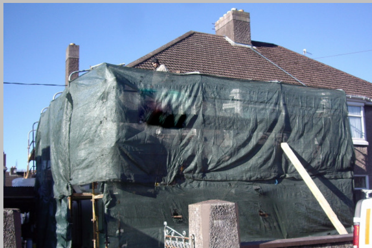
Step 6 Protect the newly rendered façade until set and dry, this will be 2-3 days approx in normal weather conditions.
