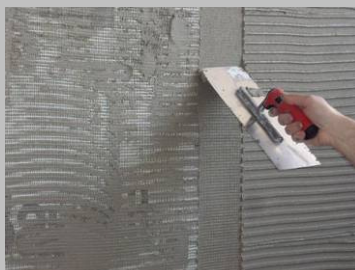
Step 7 Press the edge of the mesh sheet a little deeper into the mortar with the tip of the trowel.
