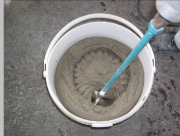
Fig. 1 Sprinkle the dry powder adhesive into clean water. Mix with an electric hand mixer at slow speed setting to a smooth, workable mortar.
