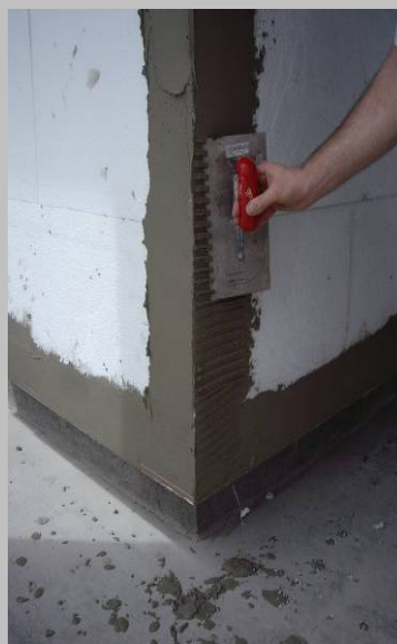
Step 5 Apply a full bed of mortar approx 150mm wide and comb through with a notched trowel to set the depth for the angle bead.
