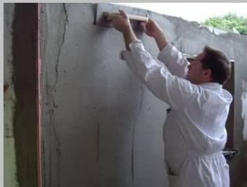
Step 3 Spray or hand apply the bonding mortar over the surface and smooth out with a trowel or plastering rule.
