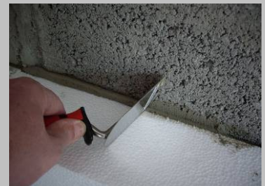
Fig. 8 Remove excess adhesive mortar
