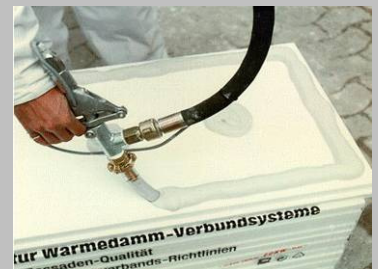
Fig. 4 A direct mix and application from a mortar pump with a pistol attachment speeds up the application of the adhesive mortar to the board.
