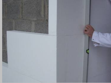
Fig. 9 Check that the boards are plumb and in line. Do not bang the boards.
