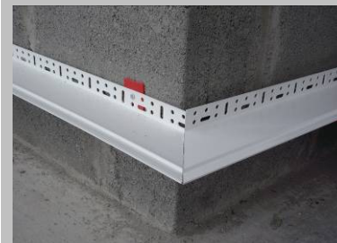
Step 8 Line up the angled cuts to form the corner.
