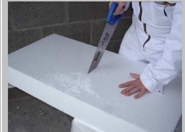
Fig. 10 EPS insulation boards can be cut with a hand saw, a "hot knife" or a "hot wire".!
