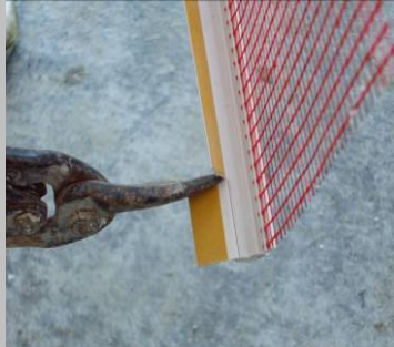
Fig.1 Measure and cut the seal beads for the vertical reveals first.
