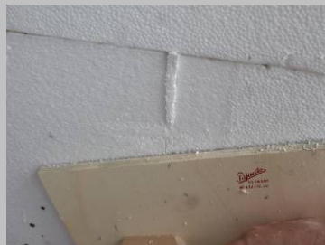
Fig. 15 Rasp back the surface of the insulation boards, removing all undulations leaving a smooth flat surface.
