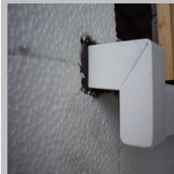
Step 6 The Expander band is there to waterproof the junctions between the board and solid objects and it therefore must be fitted tightly..
