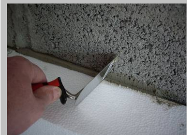
Fig. 8 Remove excess adhesive mortar
