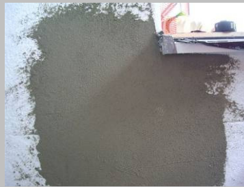
Step 1 Apply reinforcing mesh strips (min. 250 x 250mm) diagonally across the opening corners into a tight coat of bonding mortar.
