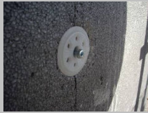
Step 3 Place the fixing head flush on the surface.
