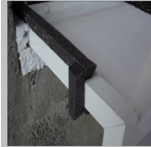
Step 4 Only apply enough band required as it will expand quickly once off the roll. Fully expanded band will be more difficult to compress later.
