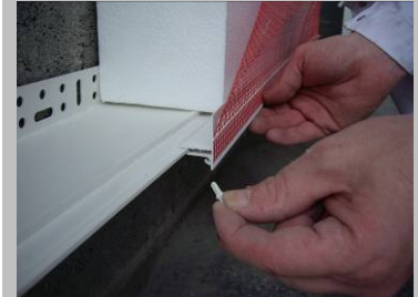
Step 10 Insert a plastic pin connector into the clip-on trim.
