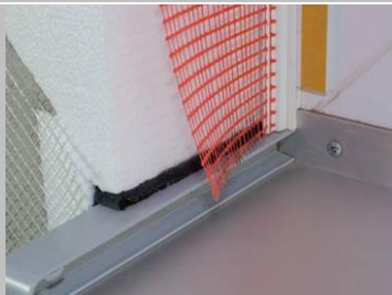
Step 5 Peel off all the yellow paper tape from the protection strip to expose the sticky surface to allow the application of polythene sheet to protect the window from mortar splashes.
