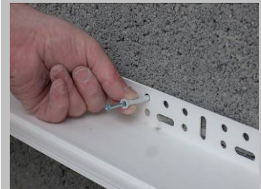
Step 2 Push the screw fixing through into the bore hole just tight enough to support the L-section.
