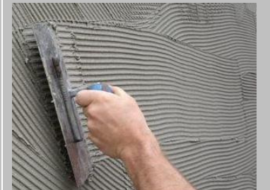
Step 4 Comb through the mortar with a notched trowel to set a uniform depth of thickness.
