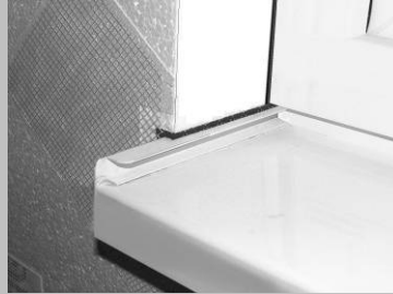
Step 1 Clean the building element to ensure the joint seal band will stick.
