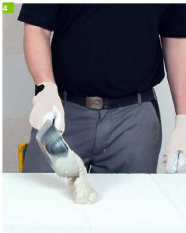
4 Apply lightweight mortar
