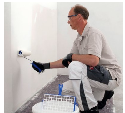
Application of Multipor interior silicate paint
