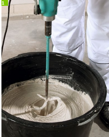
1 Mixing Multipor lightweight mortar with Multipor hemp felt insulation strips
