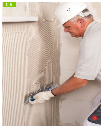
15 Apply the reinforcement layer
