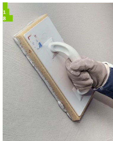
18 Felt off finishing render if necessary
