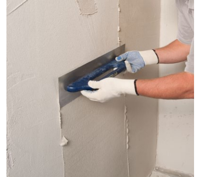
Multipor lime smoothing compound (FINISH GP830) Applying the finishing render
