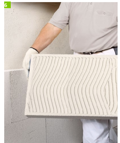
6 Full-surface mortar on mineral insulation board
