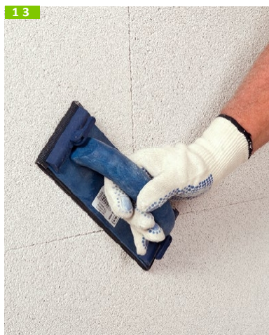
13 Sand down unevenness, sweep off sanding dust and prime if necessary
