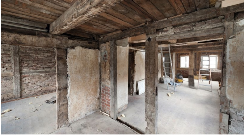
Complete core refurbishment with the Multipor WI clay interior insulation system
