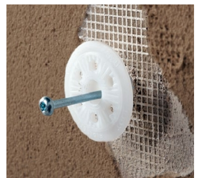
Inserting the dowel through the fabric
