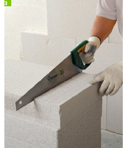
3 Cutting Multipor mineral insulation board
