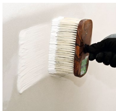
Painting the Multipor interior silicate paint
