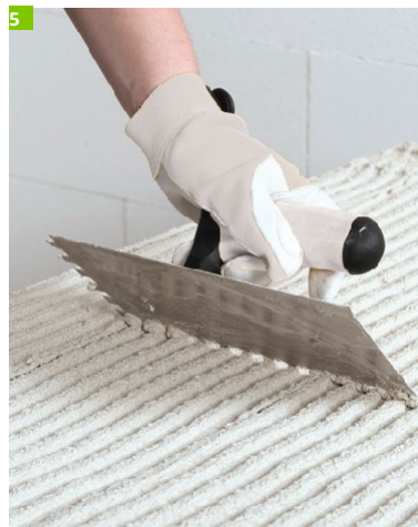
5 Comb through light mortar
