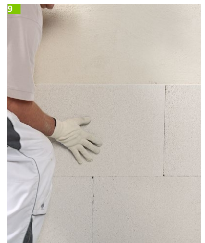
9 Butt joint and bed joint tightly butted
