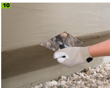
Remove the reinforcement layer and allow to dry for 24 hours
