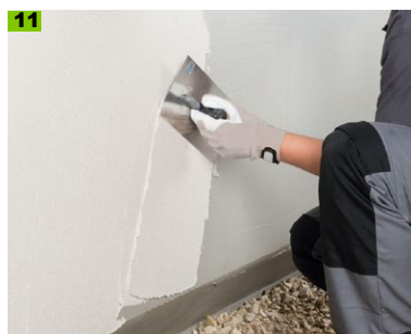
Apply finishing plaster
