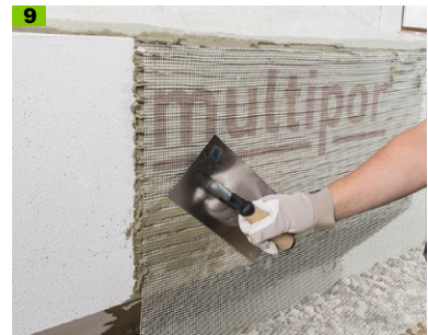
Apply Multipor reinforcing mesh and plaster in place
