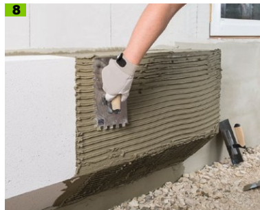
For the reinforcement layer, apply Multipor sealing slurry to the Multipor plinth insulation board
