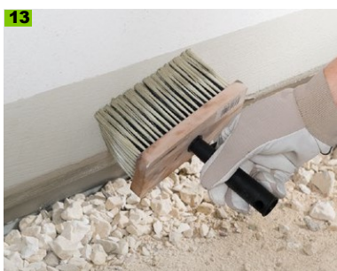
Re-coat the area of the finishing render in contact with the ground with Multipor sealing slurry for moisture protection
