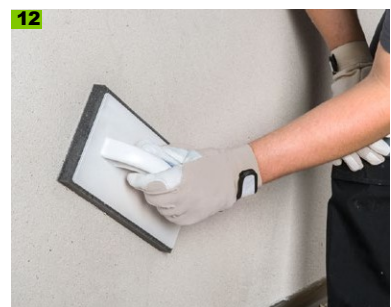
Felting or texturing finishing plaster
