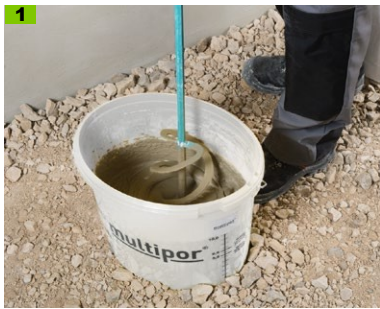
Mixing Multipor sealing slurry
