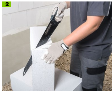
Cut Multipor plinth insulation board at an angle
