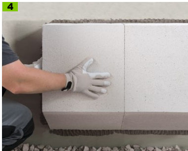
Press on Multipor plinth insulation board and float into place
