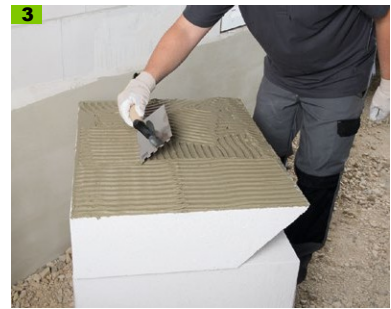
Apply Multipor sealing slurry over the entire surface with a 12 mm notched trowel
