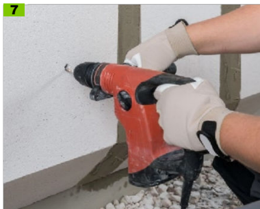
Insert Multipor screw anchors, fix Multipor plinth insulation board and leave to dry for 24 hours
