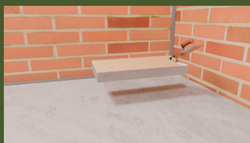
X710 Adhesive combed finish on back of Multipor Board
