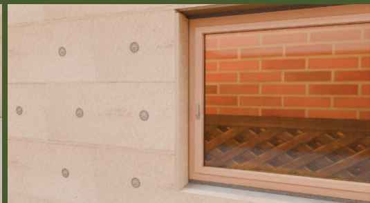
Reveal board in place pushed firmly against the Komprimax on window frame.
