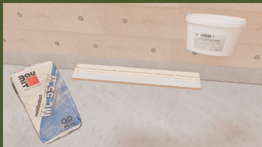
MC55 and UdiAdhesive applied to both the reveal board and to the surface of the reveal.
